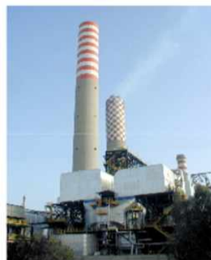
Fig. 1. 1,200,000 Nm 3 /h SNOX™ plant at the power plant of Raffineria di Gela, Italy
